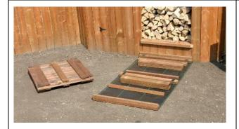
**2.** Install the 4 -2x4, 28" long foundation spreader boards between the 2 foundations sleepers that are attached to the mesh.
