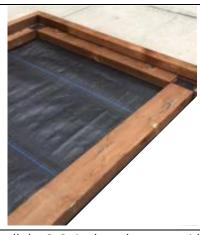
**3.** Install the 2x2 rim boards on one side using the 3" screws supplied into the pre-drilled holes
