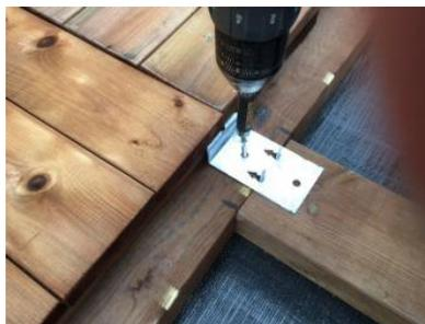
**9.** Place 3rd deck tile. Ensure tile is lined up and tight to 2 X 2 rim board. Also lined up over the 'setting prong' of the patented clip.
