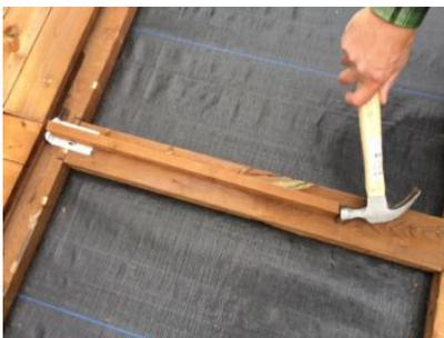
**8.** Screw down patented clip with 1 1/4 inch screws provided.
