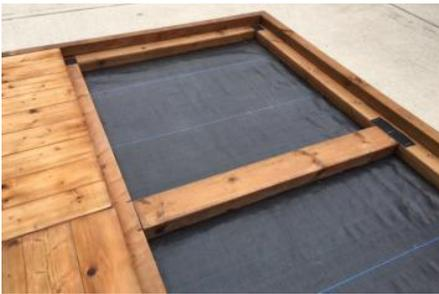
**13.** Repeating Step 7 & 8. Set and screw down patented clip with 1¼ inch screws provided.
