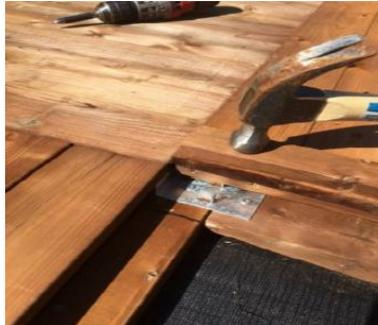
**11.** Place 4<sup>th</sup> deck tile, and repeat step 10 to also set this deck tile onto foundation using the driver board into the patented clip “prong’.
