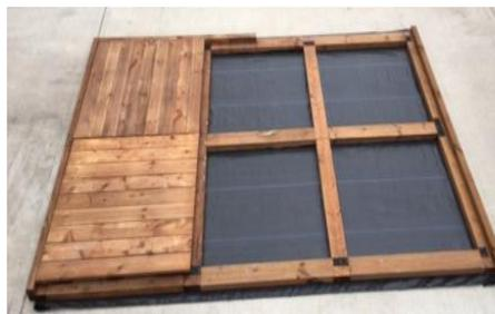
**6.** Install second 2 X 2 rim board. Place this board with predrilled screw holes facing up. Use supplied 3 inch screws.
