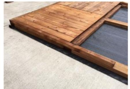
**7.** With a hammer install patented clip using 1 X 2 driver provided. Insure the tabs are driven into space between the deck tile boards. This locks the deck tile to the foundation.
