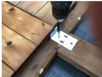
**14.** Place 5<sup>th</sup> and 6<sup>th</sup> deck tiles. Repeat steps 11 and 12 to set these deck tiles onto the foundation, using the driver board hammer into the patented clip ‘prong’
