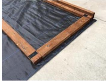
**3.** Complete installation of 9, 2 X 4-28" spreader boards as illustrated
