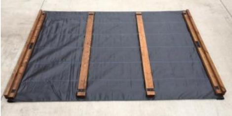
**2.** Install 2 X 4-28" long foundation spreader boards between 2 X 4 foundations sleepers
