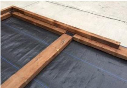
**5.** Install the first 2 deck tiles as shown. Deck tiles can be installed linear or parquet.
