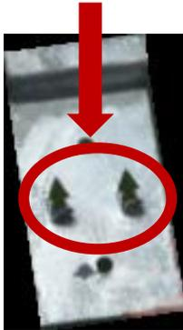
**10.** Set third deck tile into patented clip ‘prong’ by using the provided 1 X 2 driver board. You will probably need to hit the driver board several times with the hammer to set the deck tile tight to the foundation.
