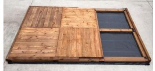
**12.** Install 3rd 2 X 2 rim board with 3 inch screws provided.
