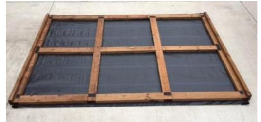
**4.** Install 1st 48" 2 X 2 rim board as illustrated, pre-drilled holes facing up, use supplied 3 inch screws.
